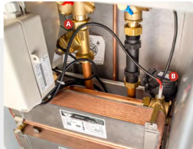
A - PICV with electronic modulating actuator
